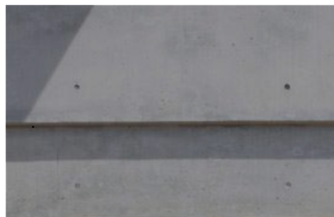
CPC3 Decorative profile finish concrete precast spandrel, material and finish to match BAL2
