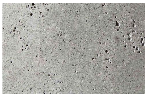
COF1 Off form Concrete with natural finish. Penetrating Clear matt sealer over
